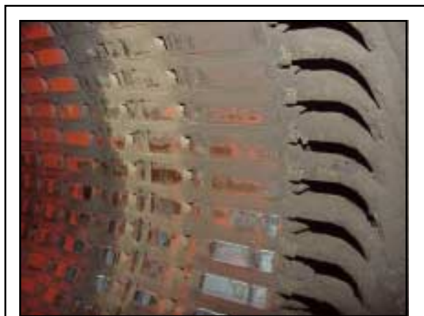
Figure 18. A minor stator core rub.
