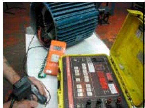
Figure 30. Measuring the resistance of a coil group. Note that meter leads are clamped securely to bare conductors; also note the ambient temperature thermometer.
